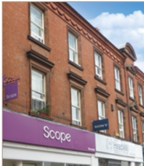
2014 - 16/17 St. Swithin's Street 6 one bedroom flats
