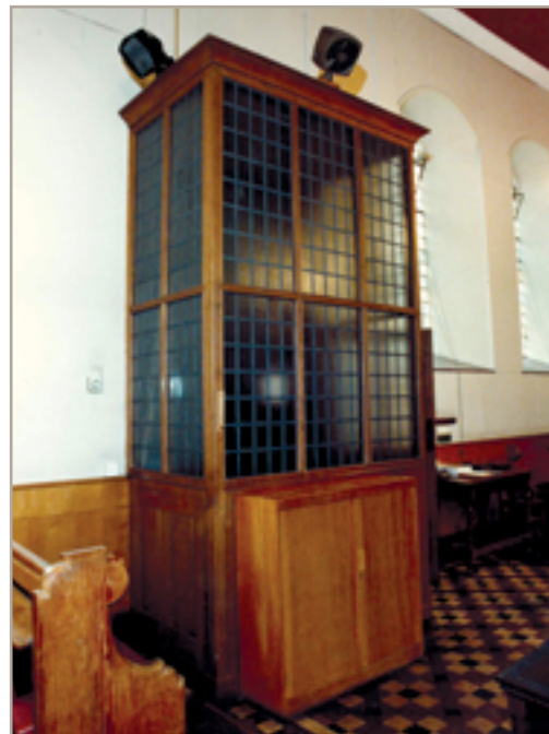
The porch to the door in 1994 with noisy electric fan heaters on top
