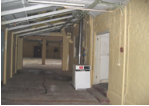
The central entrance area
