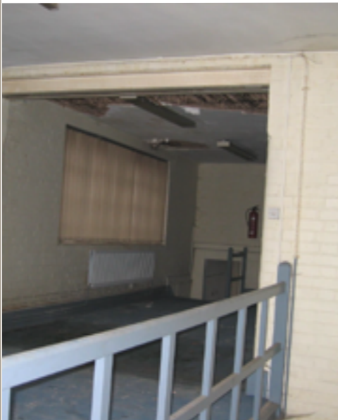
The introduction of an atrium within the heart of the building provides both natural ventilation and light into the central circulation area.
