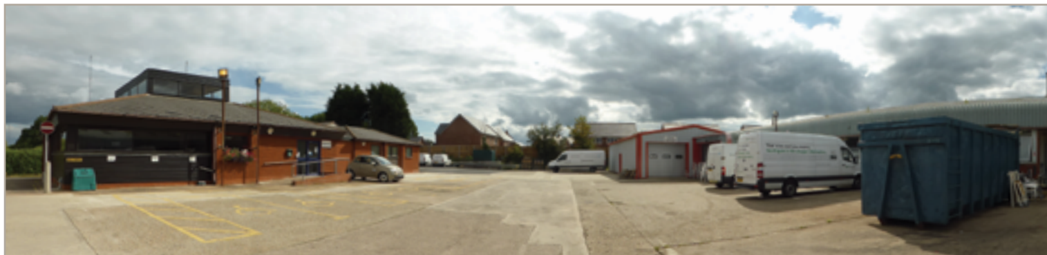
Crown Lane, showing the extent of the current site
