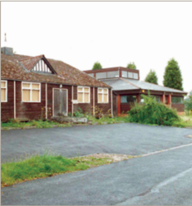
The old Village Hall was demolished
