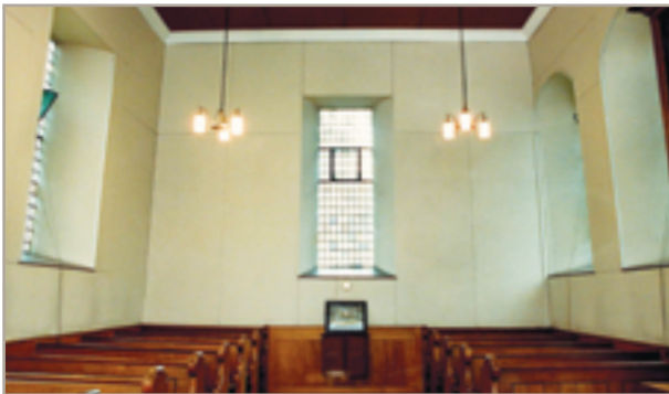
The rear of the chapel in 1994 before the door to the kitchen area was created. Note the false ceiling which was removed and the window which was reduced in size to make space for the new door
