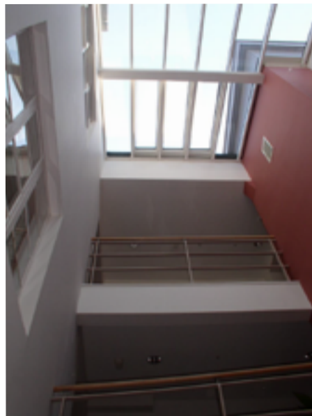
The existing building fabric, and structure, including original casement windows were retained wherever possible and repaired where necessary. Wall linings and suspended ceiling systems were used to safeguard and minimise disruption to the original building elements.
