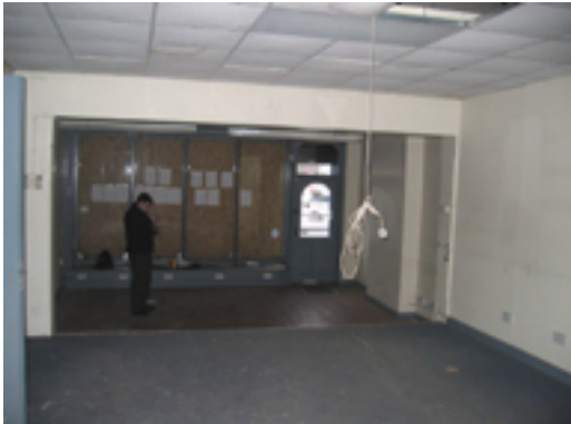
The shop front to Lowesmoor
