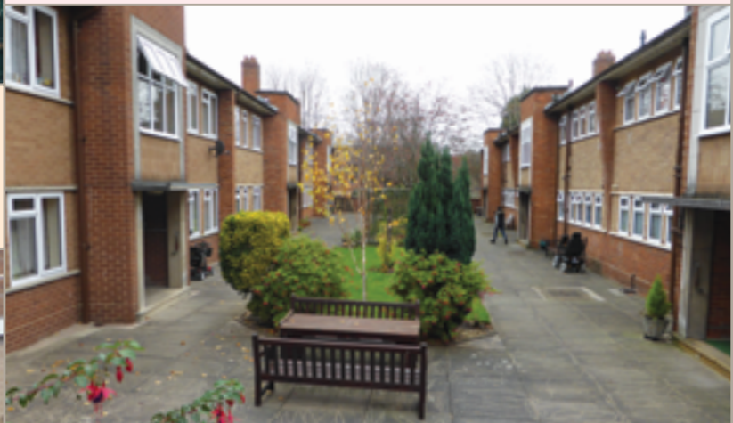
Throckmortons/Frogmortons now Nash's and Wyatt's Almshouses first described in 1531/2 as "Thorgmortons Almys hous" next to the tenement of Thomas Walker. They received bequests from the wills of James Jordan in 1525 and Robert Youle in 1561. They were apparently still in use in 1623. The site was bought by John Nash In 1639 from Brome Whorwood of Sandwell, Staffs. They then comprised 'fourteen cottages, more or less, with the little gardens thereunto..' which were pulled down and rebuilt in 1664. They were condemned as uninhabitable and rebuilt again in 1959/60. Wyatt's 6 almshouses in Friar St were also condemned as uninhabitable and 4 Wyatt's Almshouses were rebuilt on the Nash's site in 1964 and the whole was renamed "Nash's and Wyatt's".
