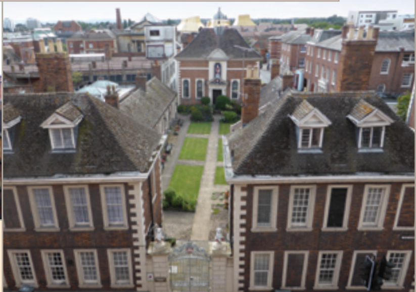
Berkeley's Almshouses and Chapel – Founded 1692 and built by 1708. Modernised twice. The first refurbishment of the Almshouses was in 1965 when each bed sitting room had a bed which was hinged to the wall. There was also a coal cupboard and sink. Outside there was a block of communal privies by the chapel. Each bedsit was given a new kitchenette, bathroom and toilet. The second refurbishment in 1981/2 when each two almshouses were turned into one, to provide separate bedrooms, kitchens and toilets.
