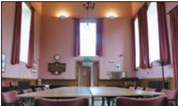
The rear of the chapel after work was completed
