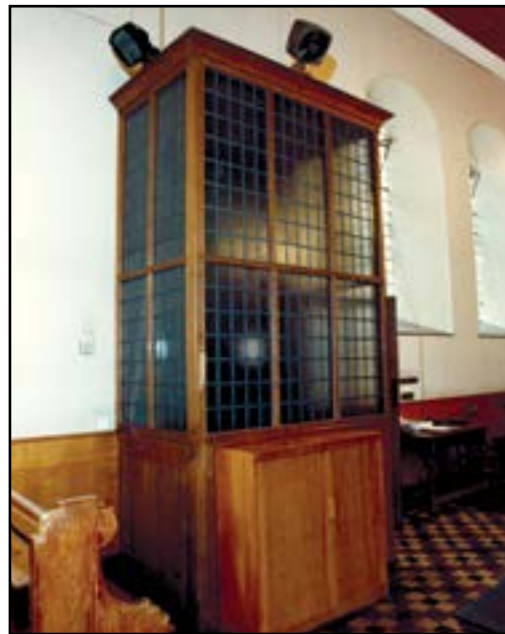
The porch to the door in 1994 with electric fan heaters on top
